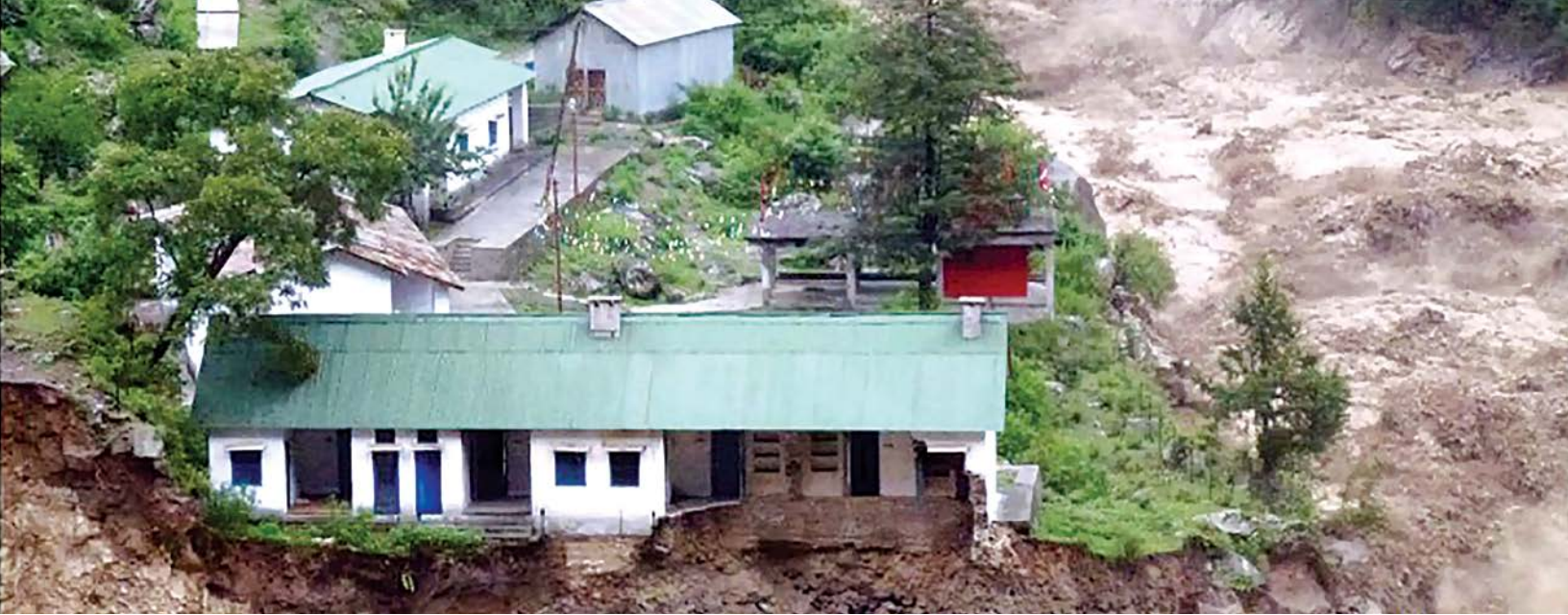
June 2013 - Buildings stand on flood-ravaged land alongside the Alaknanda River in Chamoli district, Uttarakhand (India).
